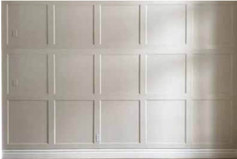
Grid pattern millwork in entry
