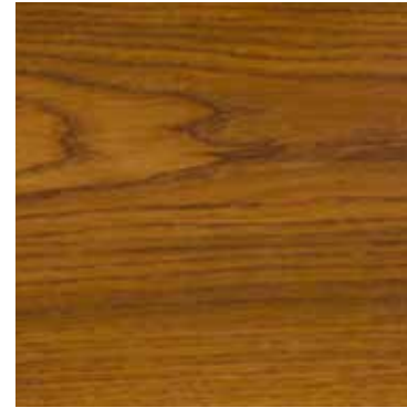
Front exterior columns and porch ceiling stain
