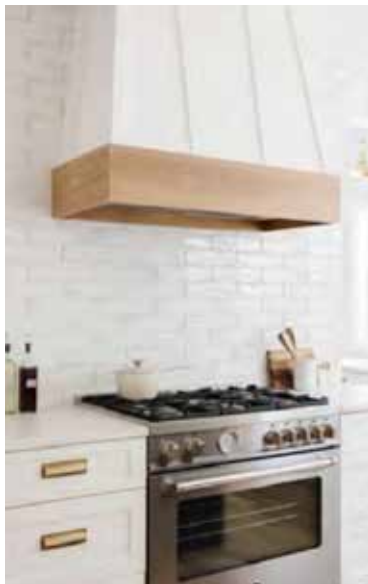
Vent hood with flat molding and white oak band at bottom
